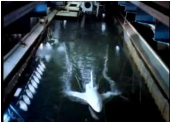
*Fig.4 1970s Space Shuttle ditching tests at Langley show lifting bodies can make safe landing on liquid.*
