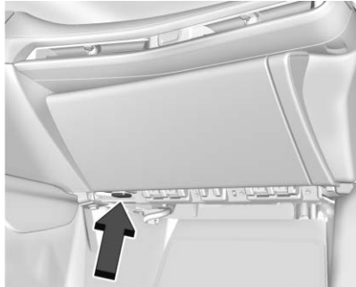
Interior Power Outlet
